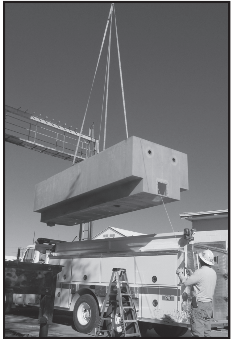
Setting back the welded water tank.
